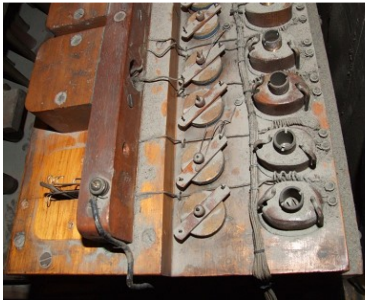
Figure 17. Double-acting slider machines at Battersea Town Hall (Copyright © Lucien Nunes)
