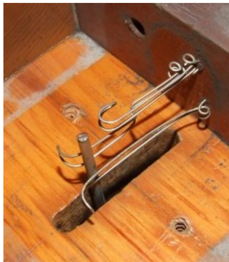
Figure 16. Automatic slider changeover switch (Battersea Town Hall) (Copyright © Lucien Nunes)
